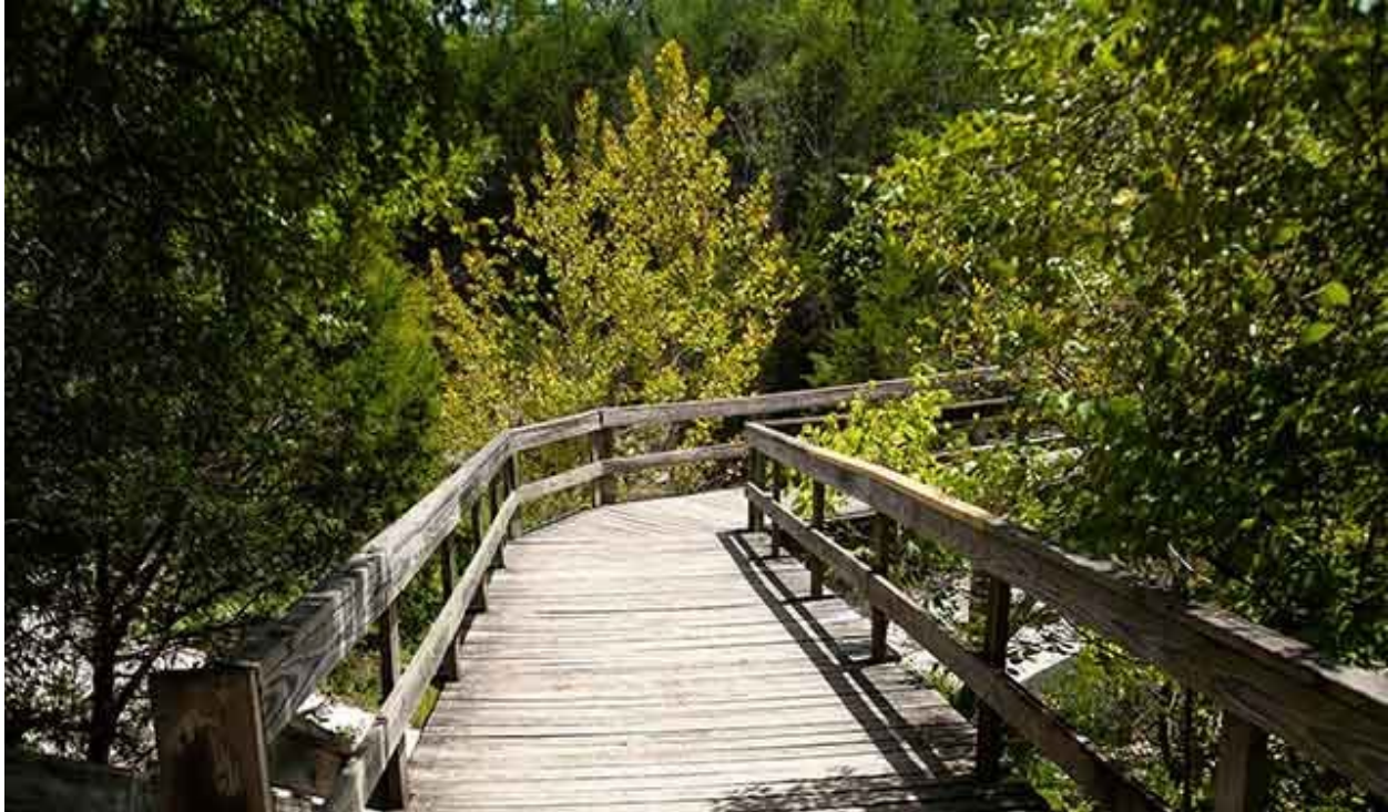
Photo 5.3 Bridge Over Gorge at Chalk Ridge Falls Environmental Center
